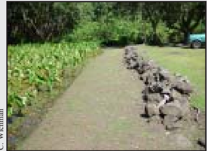
The distance from the wall to the planted area is a little over 3 feet. Note the dead tree stumps in the wall.
